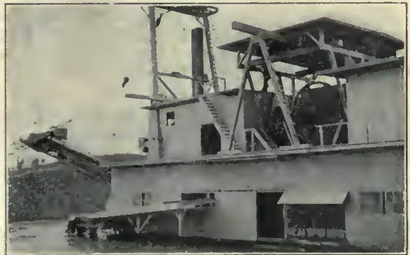
DREDGE AT OROVILLE.
